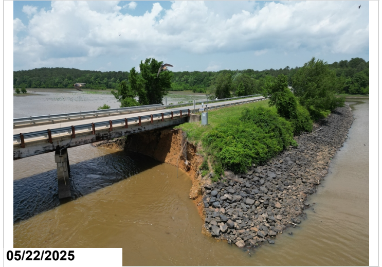
Bent 4 embankment sloughing and channel protection damage
