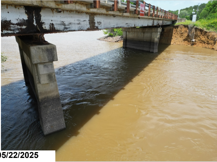
Bent 4 embankment sloughing and channel protection damage
