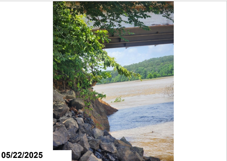
Bent 1 embankment sloughing and channel protection damage
