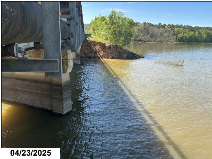
Southwest side of bridge embankment has slumped off.
