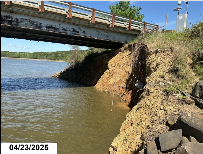
North end of bridge embankment has slumped off.
