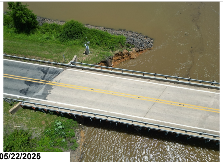
Bent 4 embankment sloughing and channel protection damage
