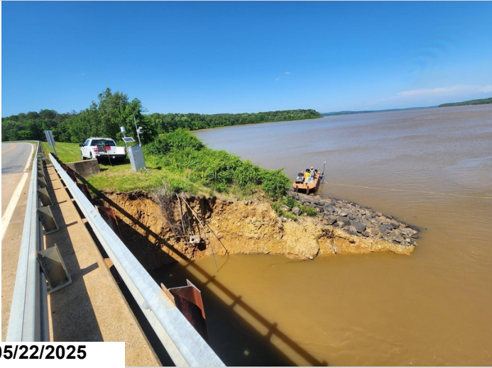
Bent 4 embankment sloughing and channel protection damage
