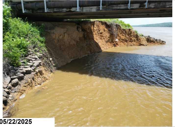
Bent 4 embankment sloughing and channel protection damage
