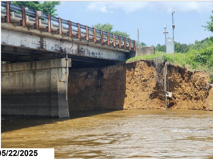
Bent 4 embankment sloughing and channel protection damage
